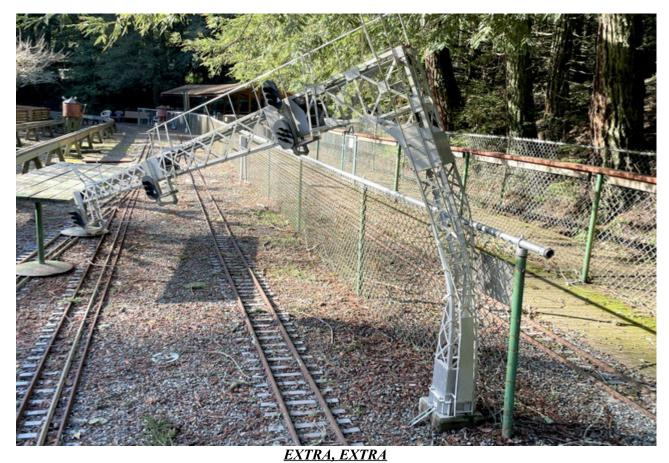
High Speed wind tearing thru the club's hill side location did this to our cantilevered signal tower! More photos inside!
