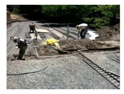
Yard trench will accept a water line and two electrical conduits to the Shattock Barn.
