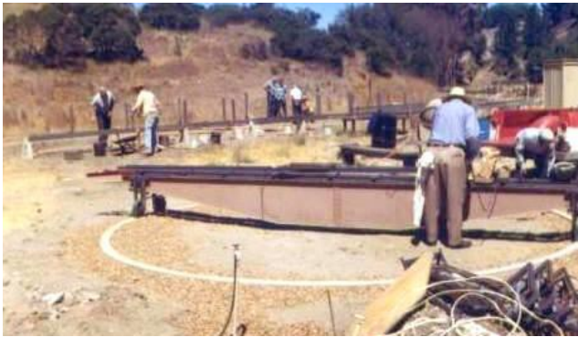
September 1972 - Construction of the turntable and elevated track continue at Tilden.
