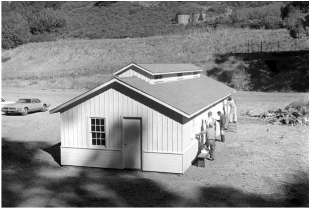
1971-ish - Our clubhouse is being finished but there are no tracks in sight. And there are two water tanks still sitting up on the hillside above the clubhouse!
