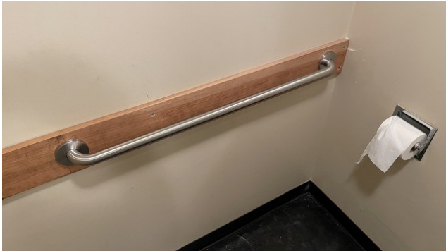
Andy Weber installed hand rails in the rest rooms and
