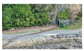
The recent earthquake in New Zealand did some substantial damage including landslides that shoved the track leading out of the tunnel into the river.
