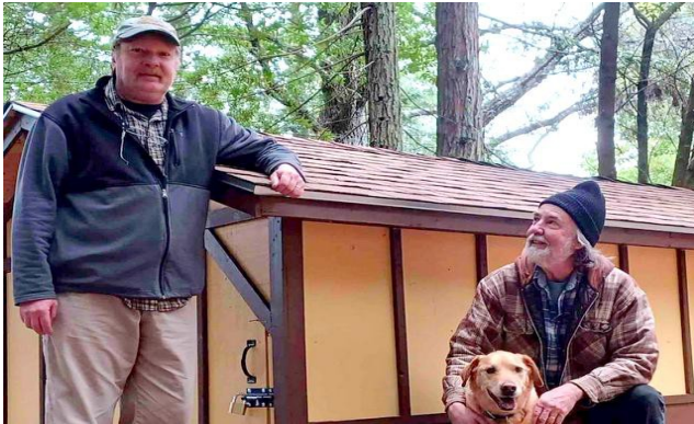
John & Wade wrap up construction on their new shed on Boyer's Bluff
