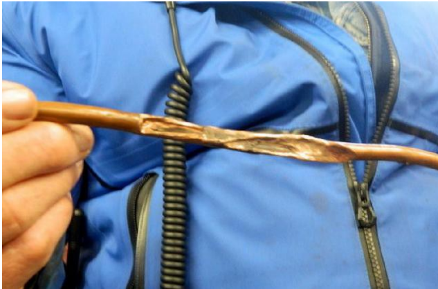
Actually, it was crushed almost flat. He paused for a brief moment to ponder if this might be the root cause of several issues, and discovered the original routing of the line positioned it to be subject to damage from the running gear. He then fabricated a new copper line and this time however, he made sure it was routed where there was no chance of a repeat occurrence. Although not fully tested at this time, Paul is confident this will solve several recent problems plaguing this engine. Thank you, Paul.
