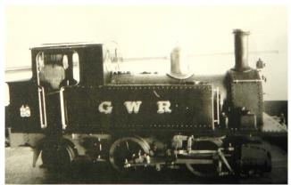
Item 1: 1.5" scale 0-4-2T locomotive, coal or wood fired, commercially built copper boiler with 200 psi hydro test certificate. Locomotive is light weight and can be moved around by two people, probably.
