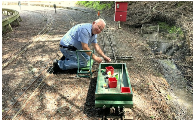
Walt doing his favorite job -- replacing signal jumpers! (photo sent in by Rich Croll)
