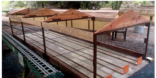
Following a long winter, work continues on the new Lisherness/Johnson/Sargent/Hirsh shed.
