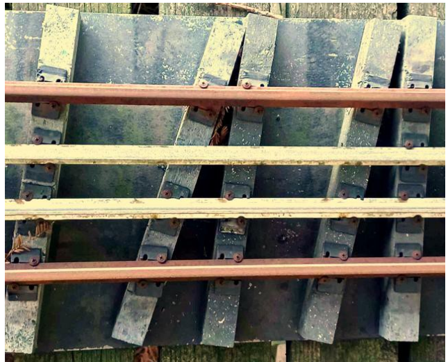
Looking to help the club? Possibly re-space ties that have been knocked out of position.
