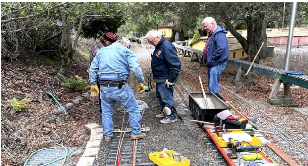
Alex O'Donnell and Paul Hirsh are leveling the first turnout while Rick Reaves and John Croll supervise
