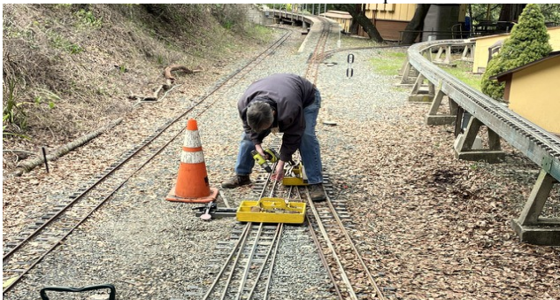
New member Jim McKibbin is finishing installing the third rail
