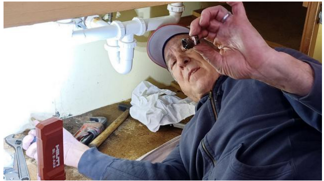
Andy Weber seen replaces the kitchen faucet.
