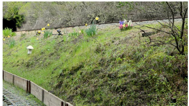
Potential land slippage by the Shattock Barn.
