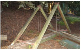
The old king post bridge from the Heinz Loop has been removed and is available for reuse. The floor stringers need replacing, but otherwise it is useable. Note it is 12 feet long and needs four individuals to carry and load it and it will be available in the parking lot at the Fall Meet. Any member who is interested should make an offer on the silent auction sheet which will be on the bulletinboard in the clubhouse. The auction will be closed at noon on Sunday, October 6.
