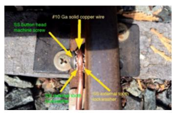
We continue to have dark block signals from the signal system logic whenever a broken rail bond wire or a loose bond connection in a section of track is detected. Derailments often damage or even break bond wires, as well they can loosen connections and/ or bend rail joint plate screws. Signal team members have collectively discussed, at some point, a newer type of rail bond (please see adjacent photos). This
