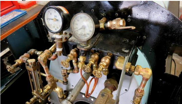
John Lisherness continues his work piping the Heinz Atlantic.
